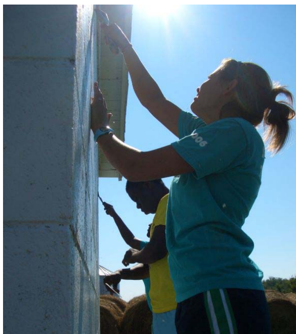
Hill Baptist works on painting our wood shop.
